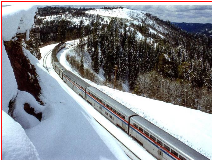
In 1991, on its crossing of Southern Pacific's Donner Pass, Amtrak's California Zephyr negotiated the narrow ledge between two chasms known as Smart Ridge, at Emigrant Gap, Calif. Surveyed in the 1860s, this 150-year-old main line runs parallel to Interstate 80.
